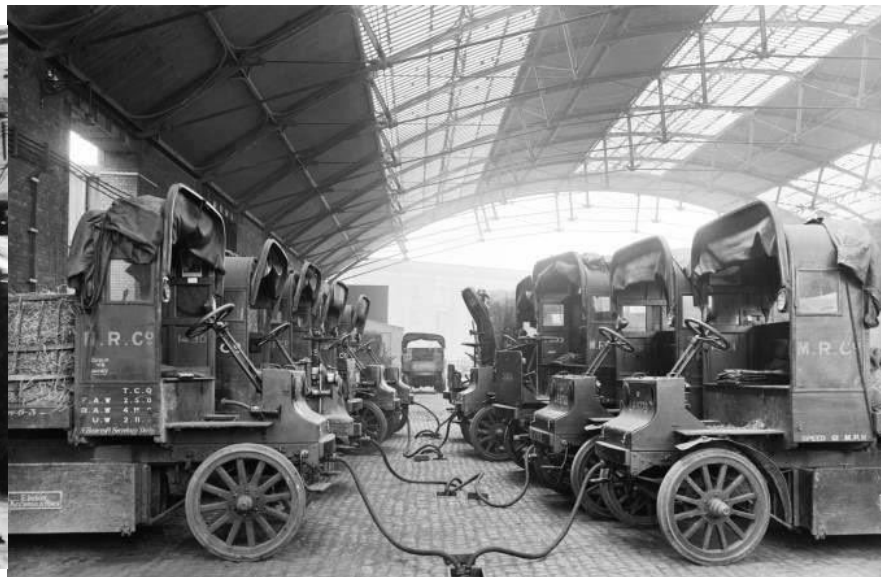
DC Charging from ground-well
