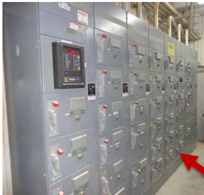
Motor Control Center (MCC) panel
