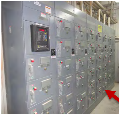
Motor Control Center (MCC) panel
